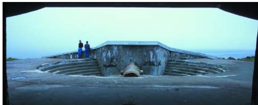
Cape Spear. The remains of a WWII battery at North America's easternmost point.
