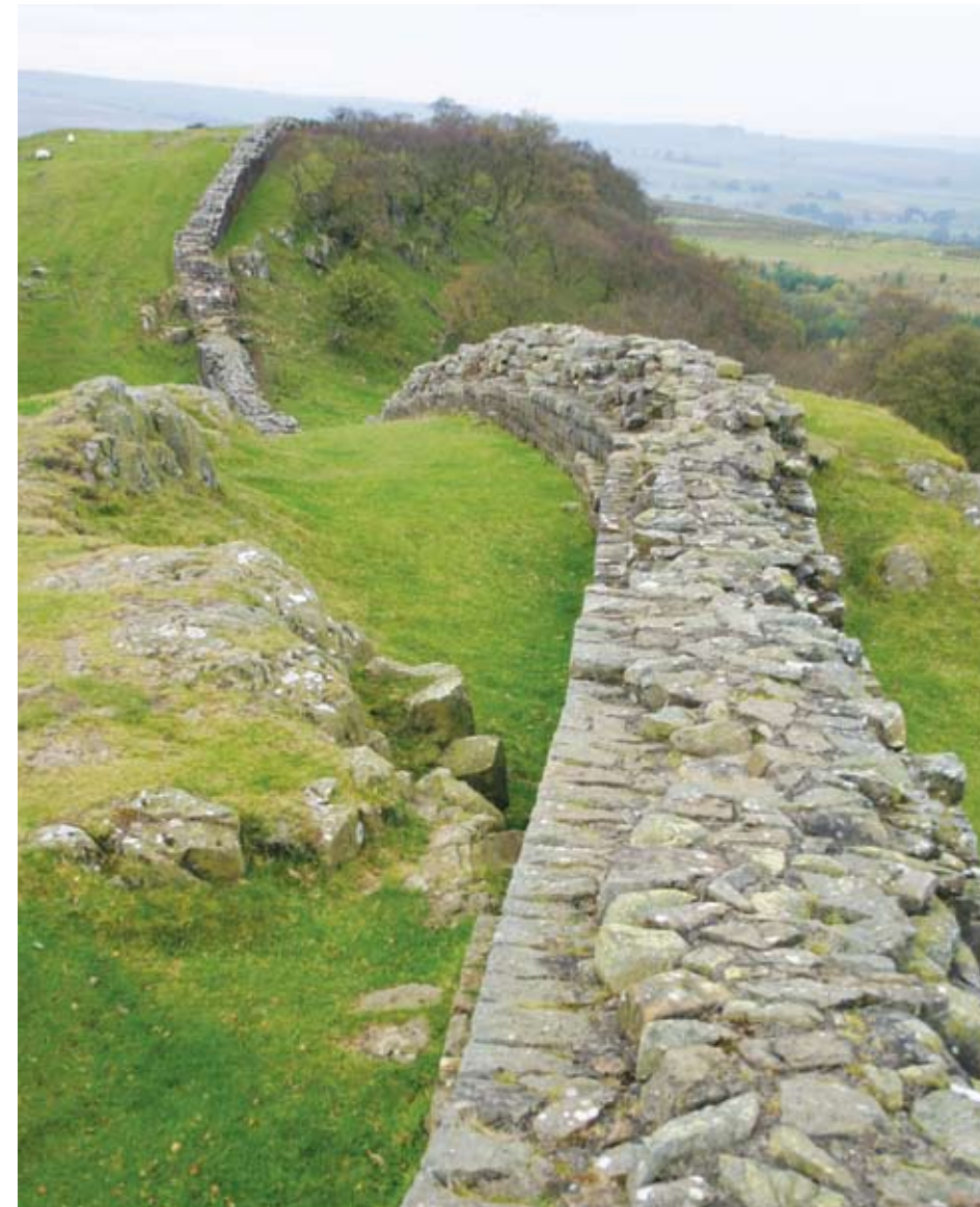
Mere remnants. A section of Hadrian's Wall at Walltown Crags near Greenhead, England.
